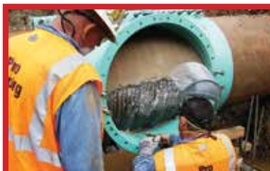
30" X 24" Wet Tap on PCCP Water Line
