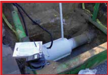
12" Pipe Freeze on DI Water Line
