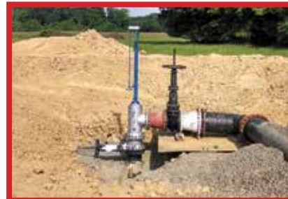
24" X 16" Line Stop on CS Sewer Line
