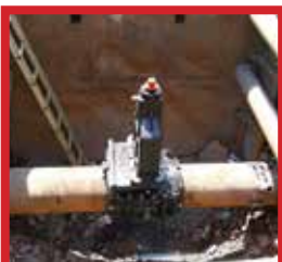
16" Valve Insertion on CI Water Line
