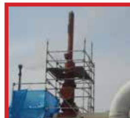
30" 150# Line Stop on CS Flare Line
