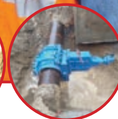
16" Horizontal Valve Insertion on DI Water Line
