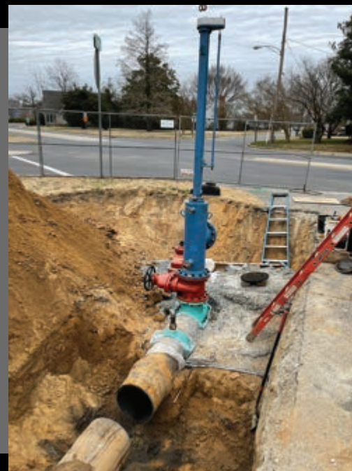
16" line stop on dip force main
