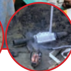
6" Pipe Freeze on DI Water Line
