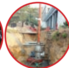
10" Line Stop on CI Water Line
