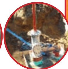
16" Line Stop on CI Water Line
